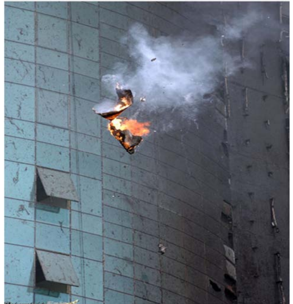
Fire spread through ACP Cladding
