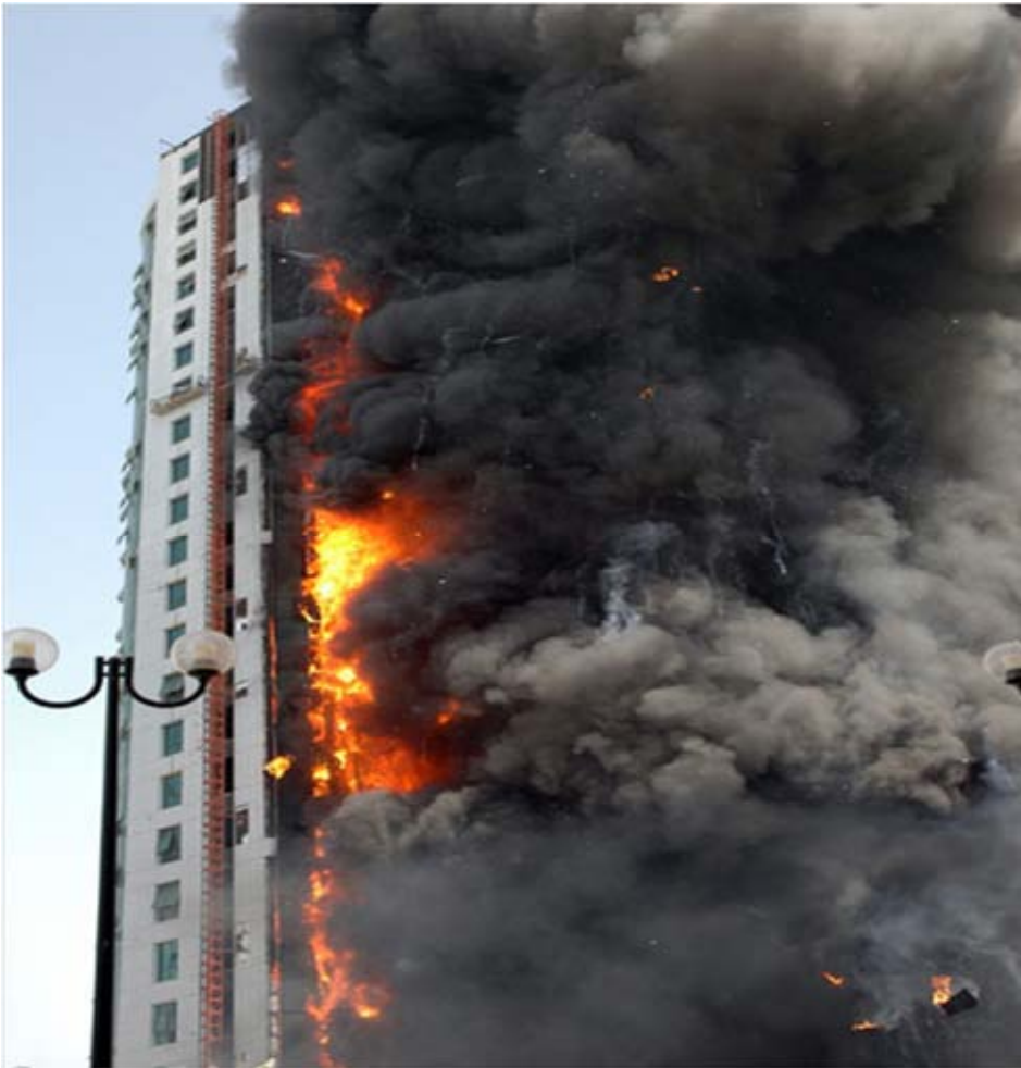
Fire spread through ACP Cladding
