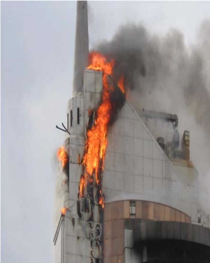
Fire spread through ACP Cladding
