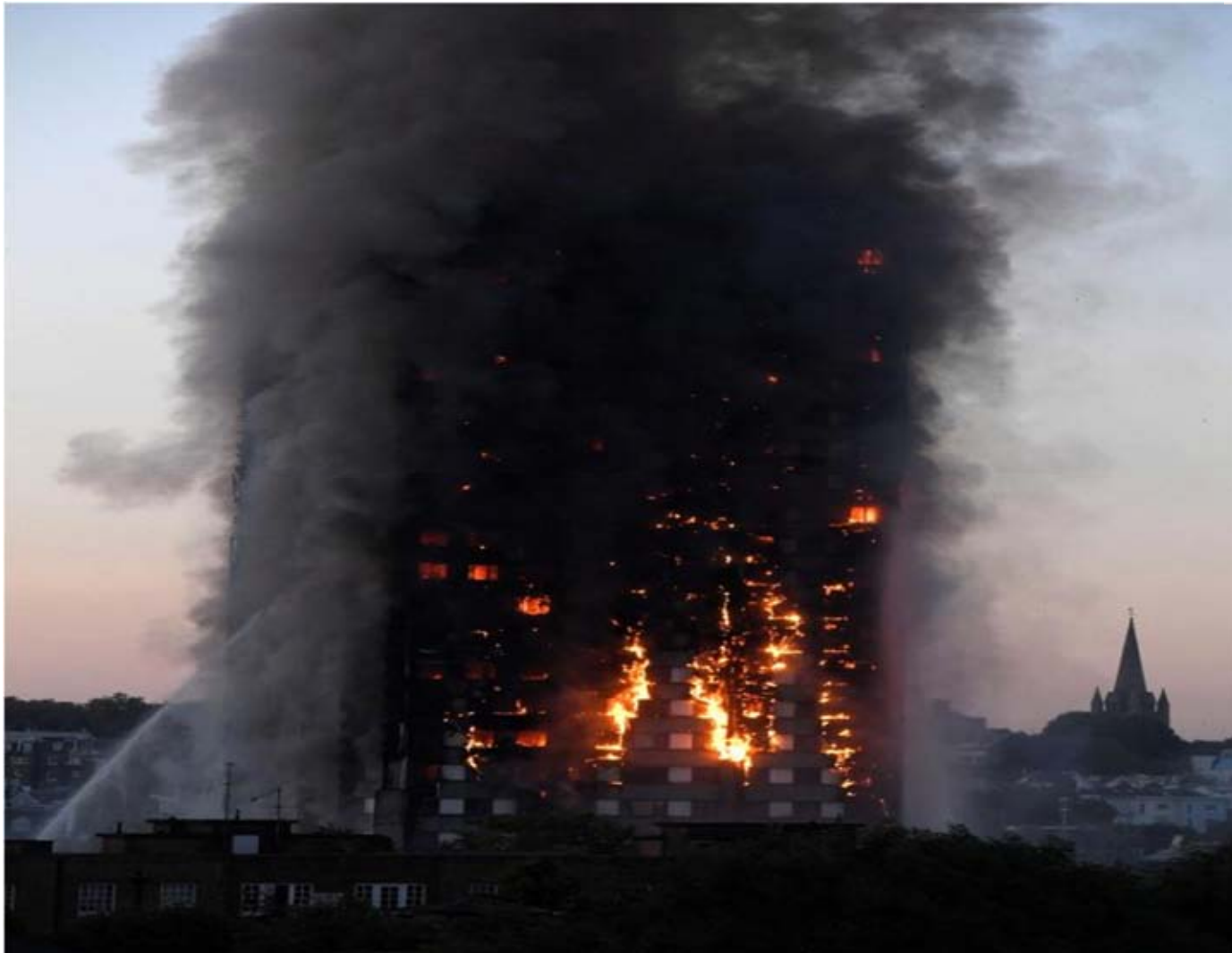
Fire spread through ACP Cladding
