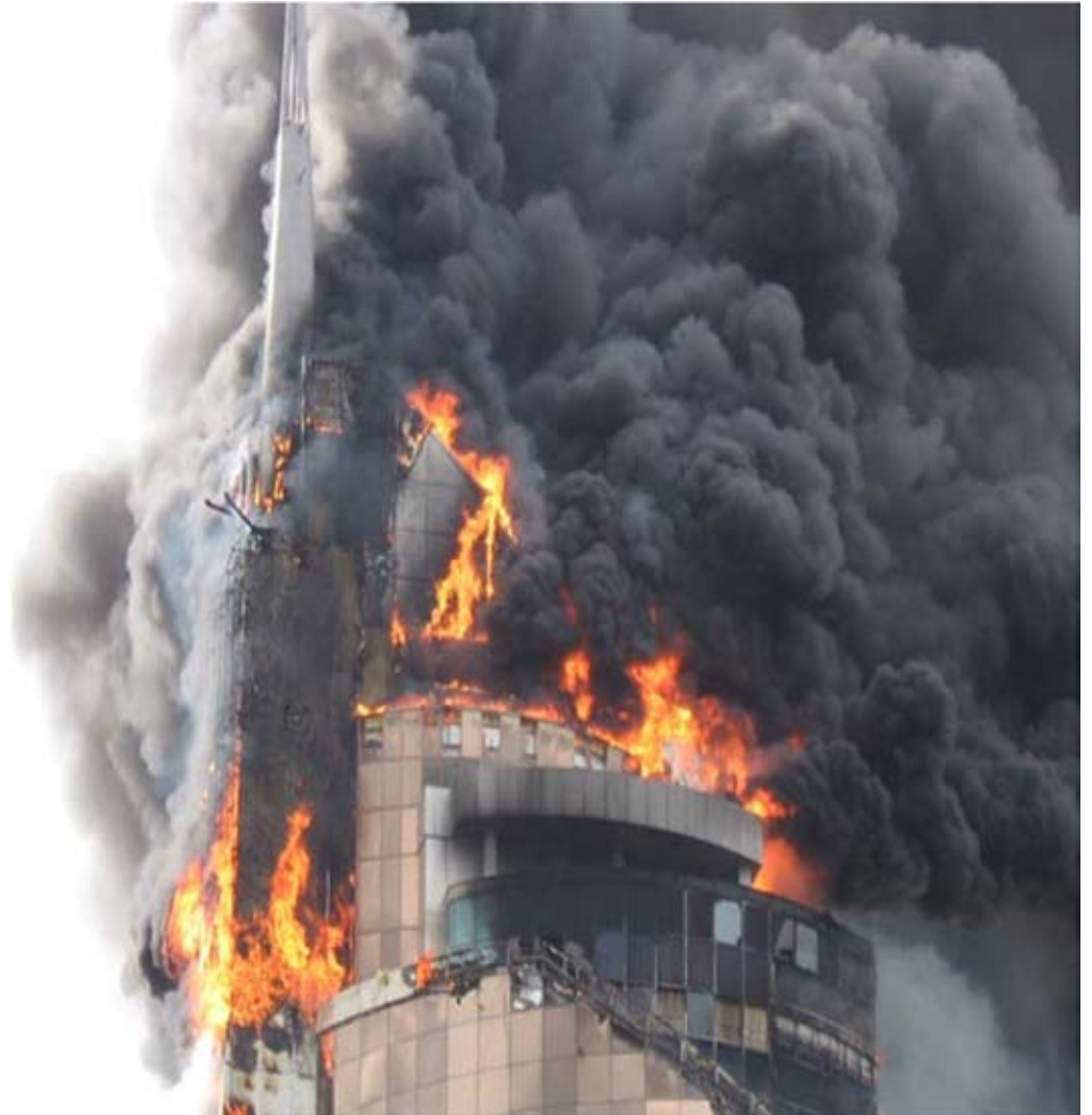
Fire spread through ACP Cladding
